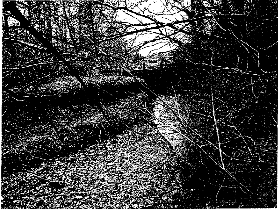
Plate D.19 View of Pendleton Brook (looking downstream) – not former flow control structure at upstream end of depot
