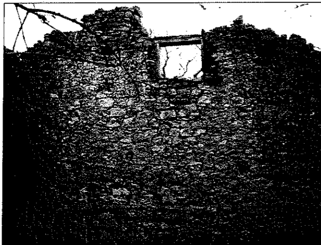
Photo 7.5 1c: Dilapidated and exposed condition of Building 1
