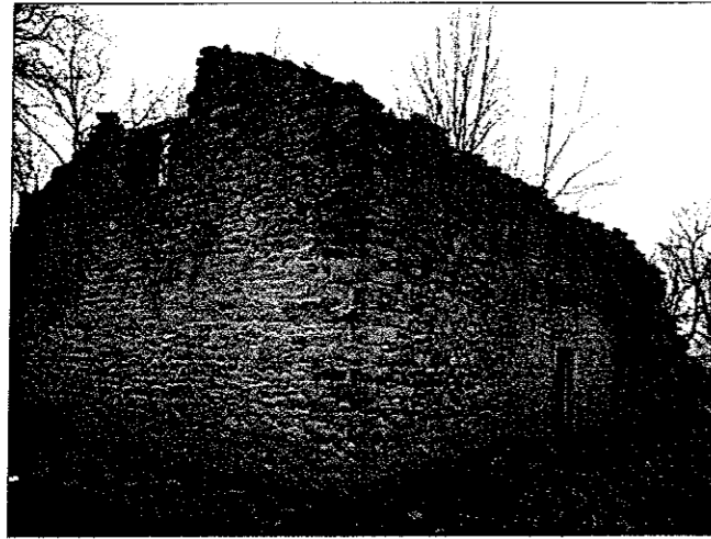
Photo 7.5 1a: Dilapidated and exposed condition of Building 1
