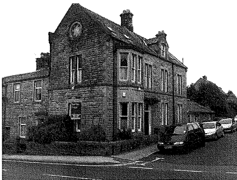
The Manse, as viewed from Berry Lane
