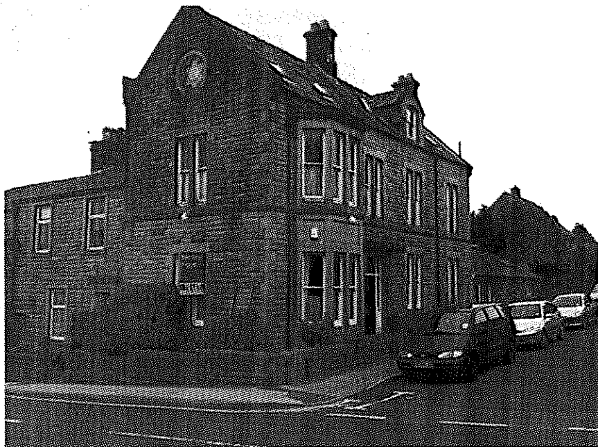
The Manse, as viewed from Berry Lane
