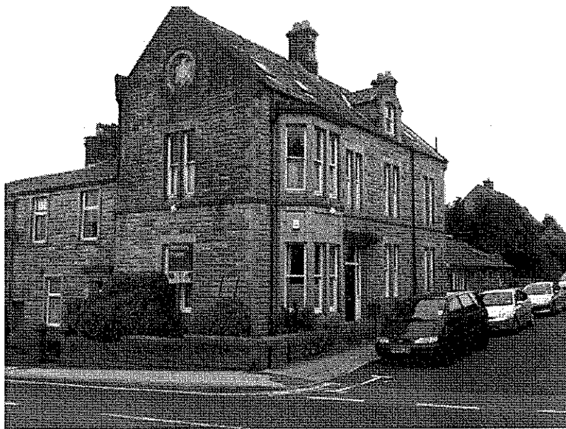
The Manse, as viewed from Berry Lane
