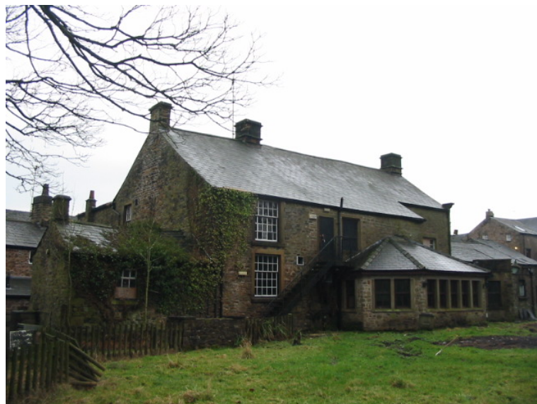
Photo 2 – View of Rear of Hotel
