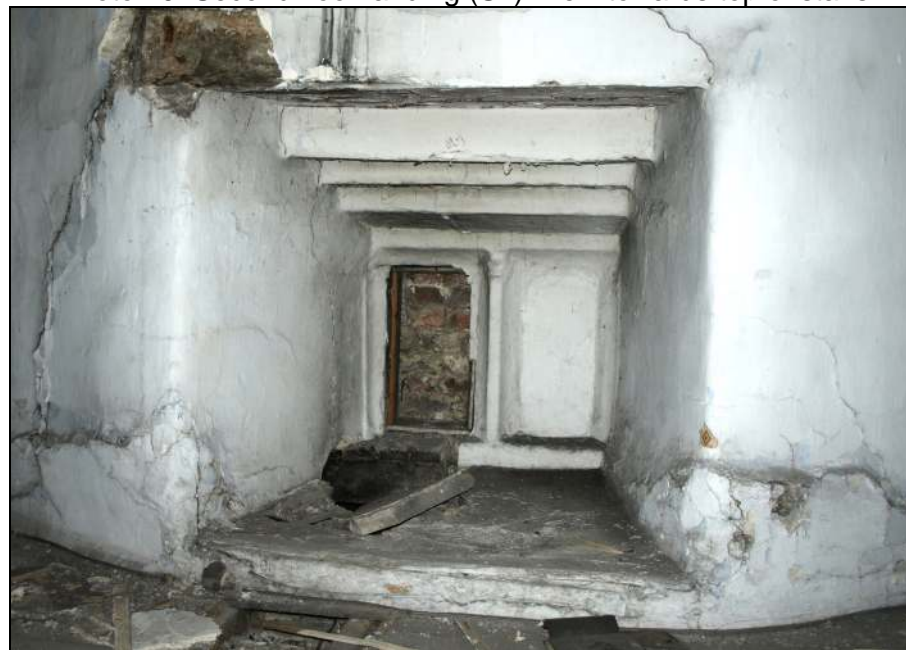
Photo 21: Blocked second floor window in north-east gable of 1779 building
