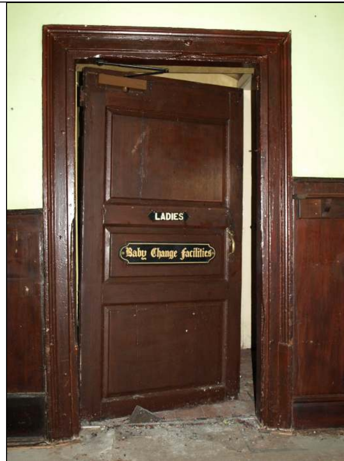
Photo 10: Original, 18th century 3 panel door to room G5 off stair hall, with intact architrave and panelling (to left)
