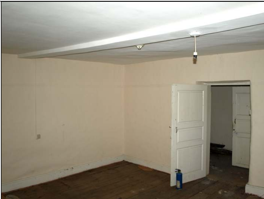
Photo 15: Bedroom on first floor (F4) with 18th century 3 panel door and plastered tie-beam
