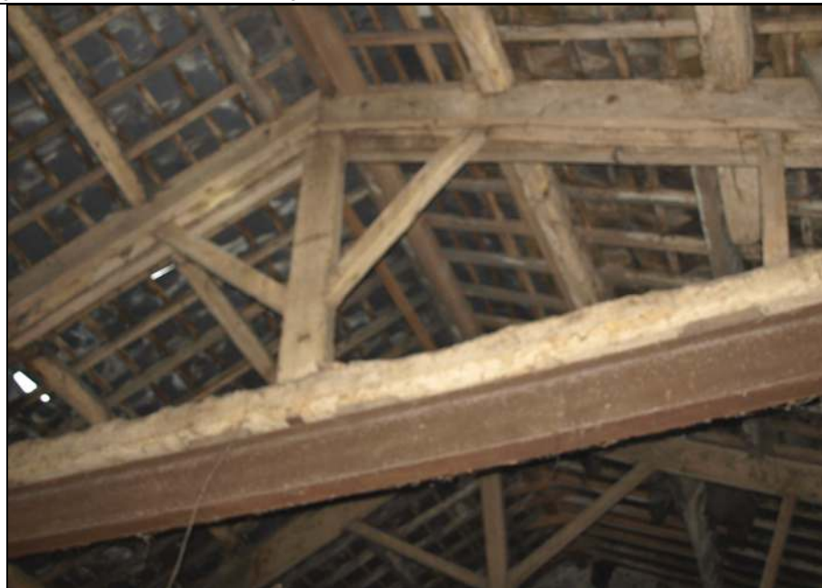
Photo 32: One of the roof trusses in the barn
