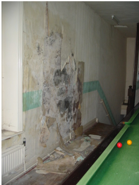
Photo 12 – Damp in Snooker Room Wall
