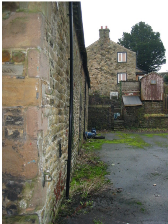
Photo 22 – Distorted Rear Wall of Barn
