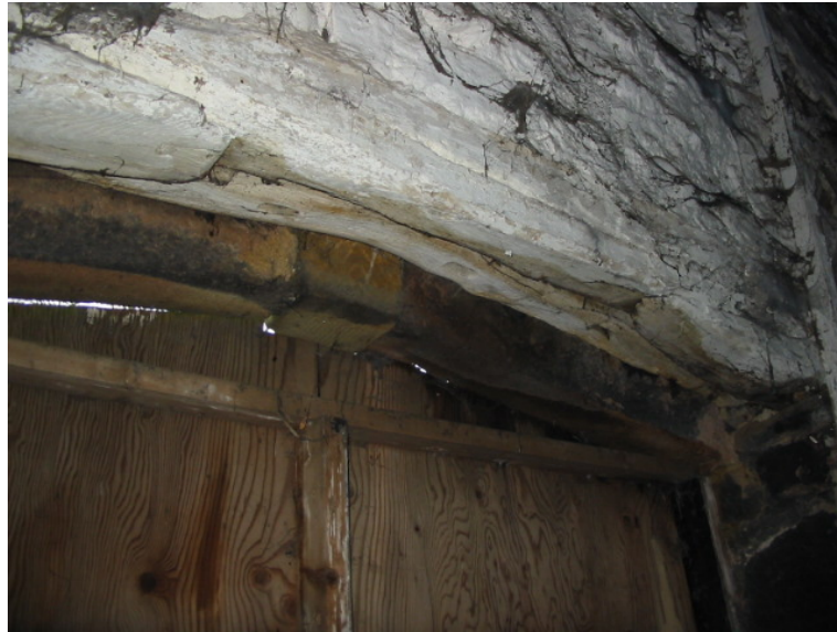
Photo 19 – Decayed Timber Lintel above Rear Door of Barn
