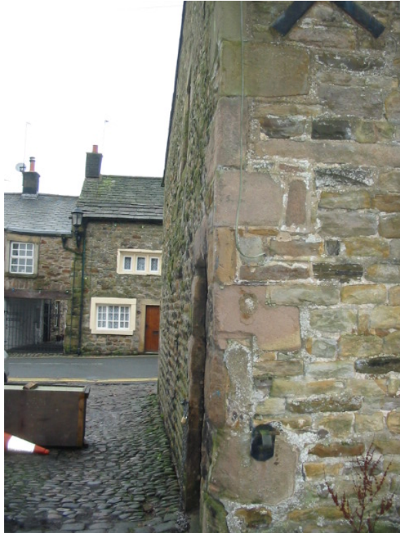
Photo 21 - Distorted Right Gable Wall of Barn
