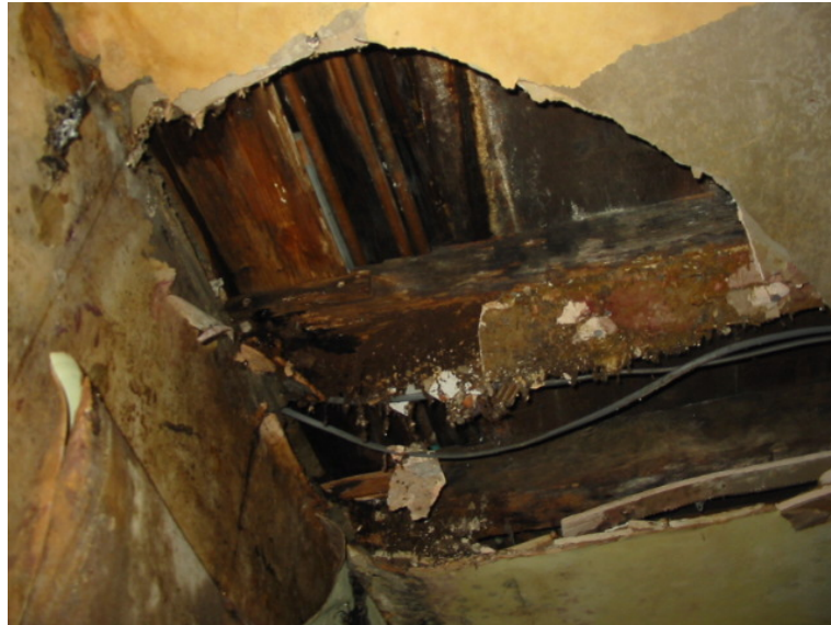
Photo 13 – Decayed Timbers - Rear Wall, Ground Floor
