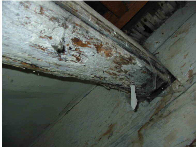
Photo 5 – Decayed Timber Purlin
