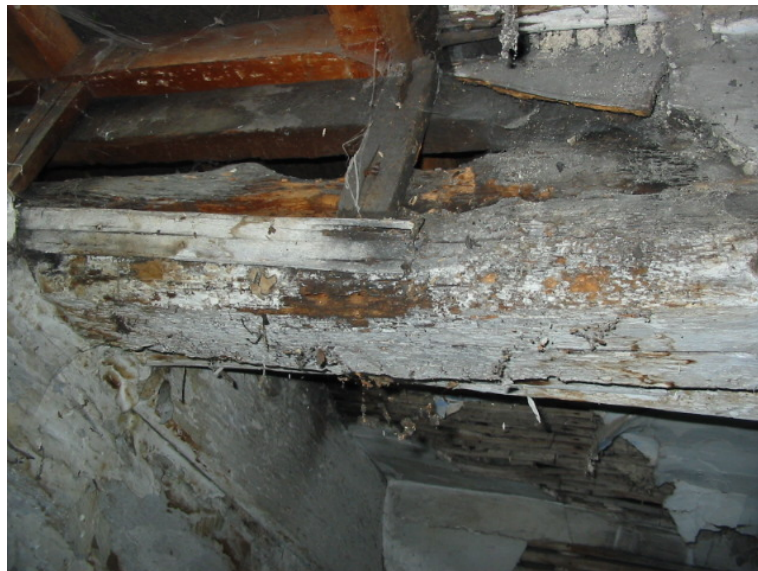
Photo 6 – Decayed Timber Purlin
