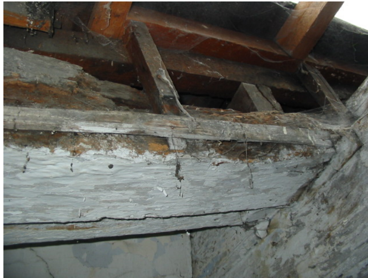
Photo 7 – Decayed Timber Purlin
