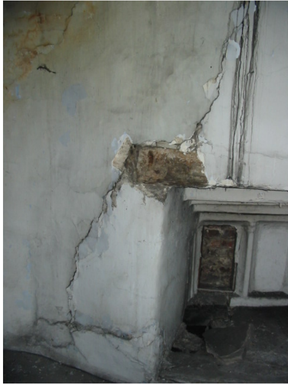
Photo 9 – Decayed Lintel and Cracking at Right Gable Wall
