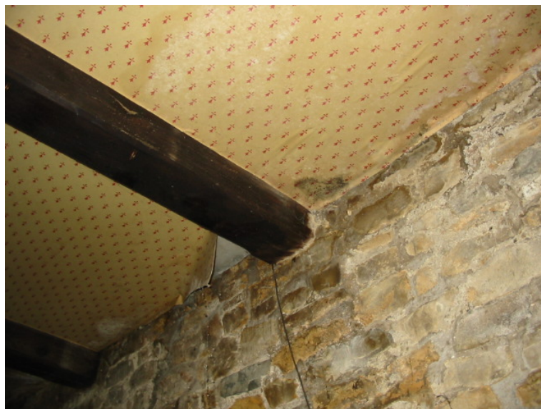
Photo 14 – Damp Staining – Left Wall, Front Lounge, Ground Floor
