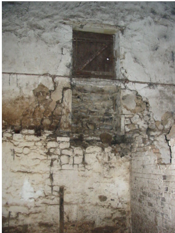
Photo 20 – Cracked and Loose Stonework on Inside of Right Gable Wall of Barn
