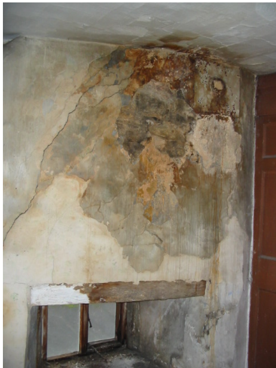
Photo 8 – Damp Staining at Left Gable Wall
