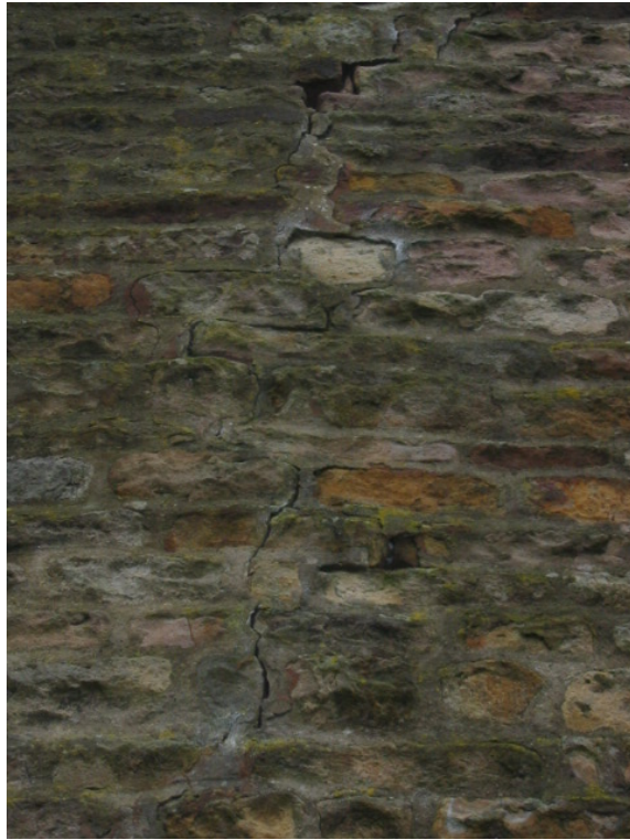
Photo 17 – Crack and Hole in Left Gable Wall
