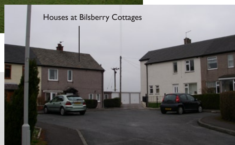
View of the houses at Bilsberry Cottages, from the northern edge of the application site
