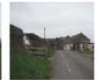
St Joseph's RC Primary School tucked behind higher landform and a hedgerow
