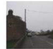
View of site corner as Whalley Road enters Hurst Green
