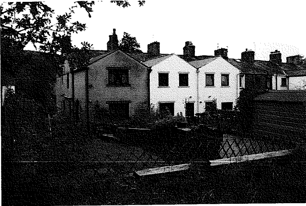
Image 2 showing two storey extensions typical of Sabden Conservation Area.
