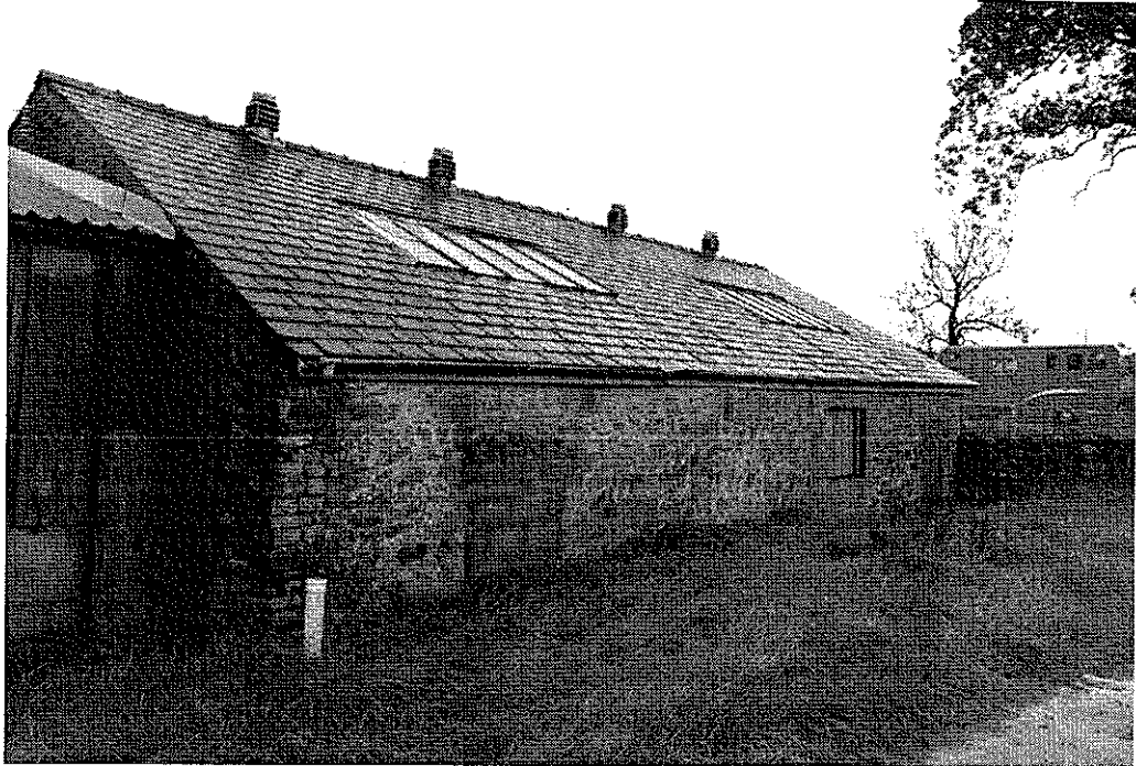
South Elevation of Goodcrooks Laithe
