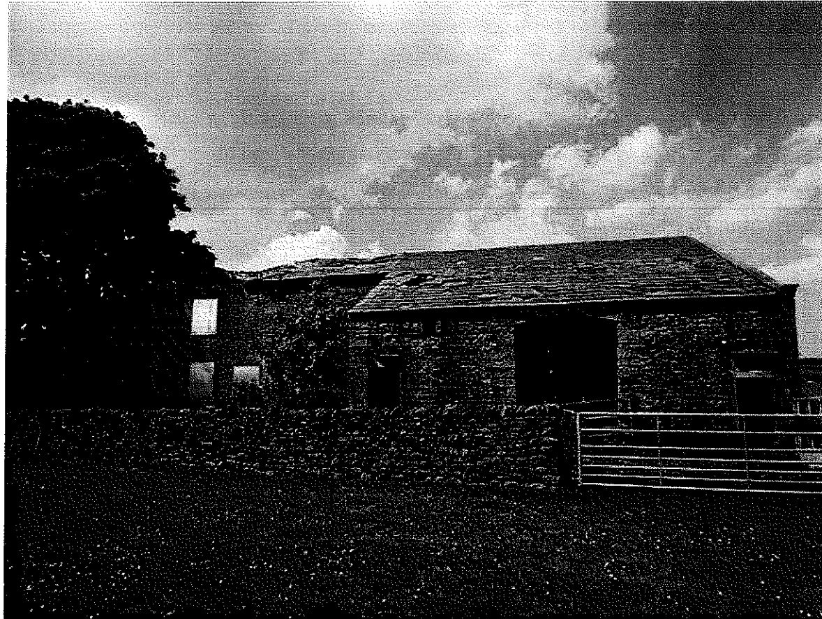
Image 1: Rear Elevation showing boarded up windows and dilapidated roof
