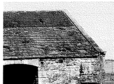
General condition of barn roof - east slope
