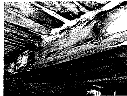
Timber decay in mistal 1 st floor
