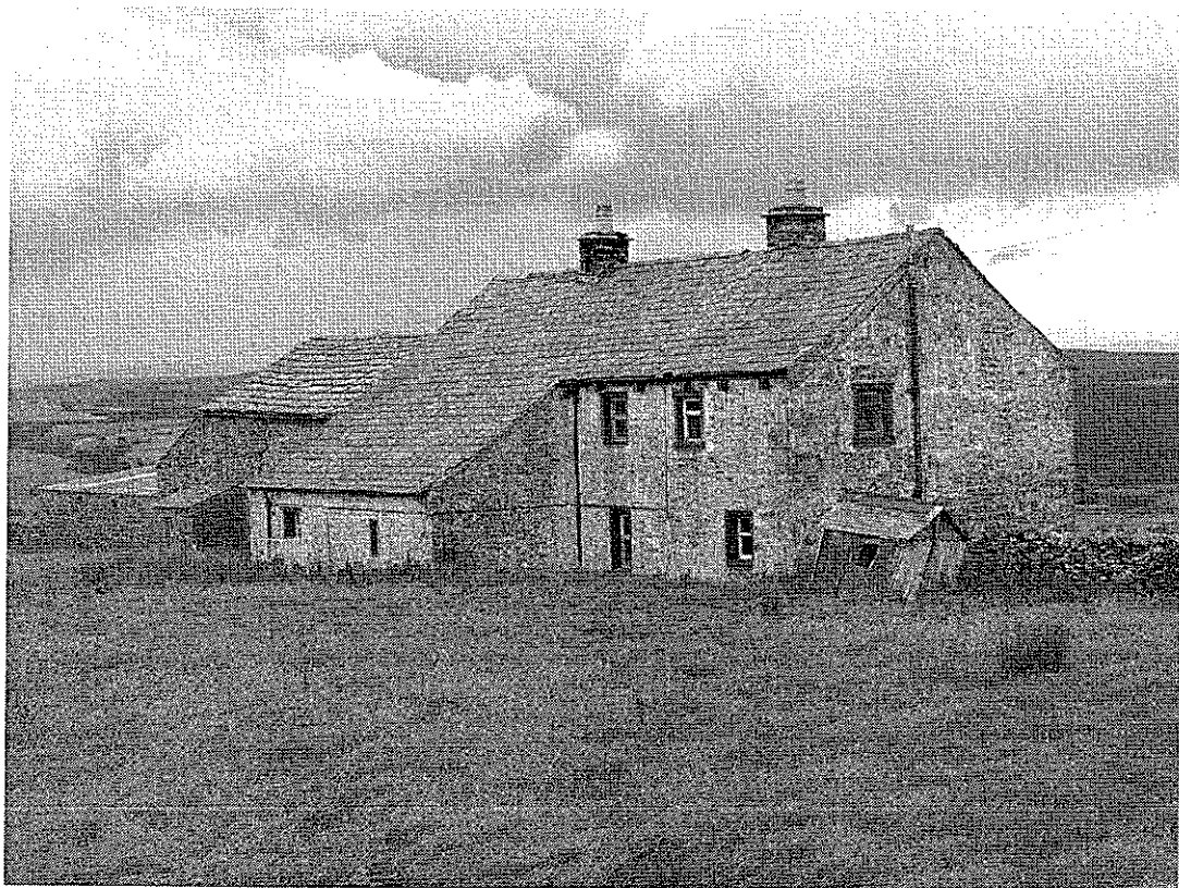
Approach to Merrybent Hill Farm
