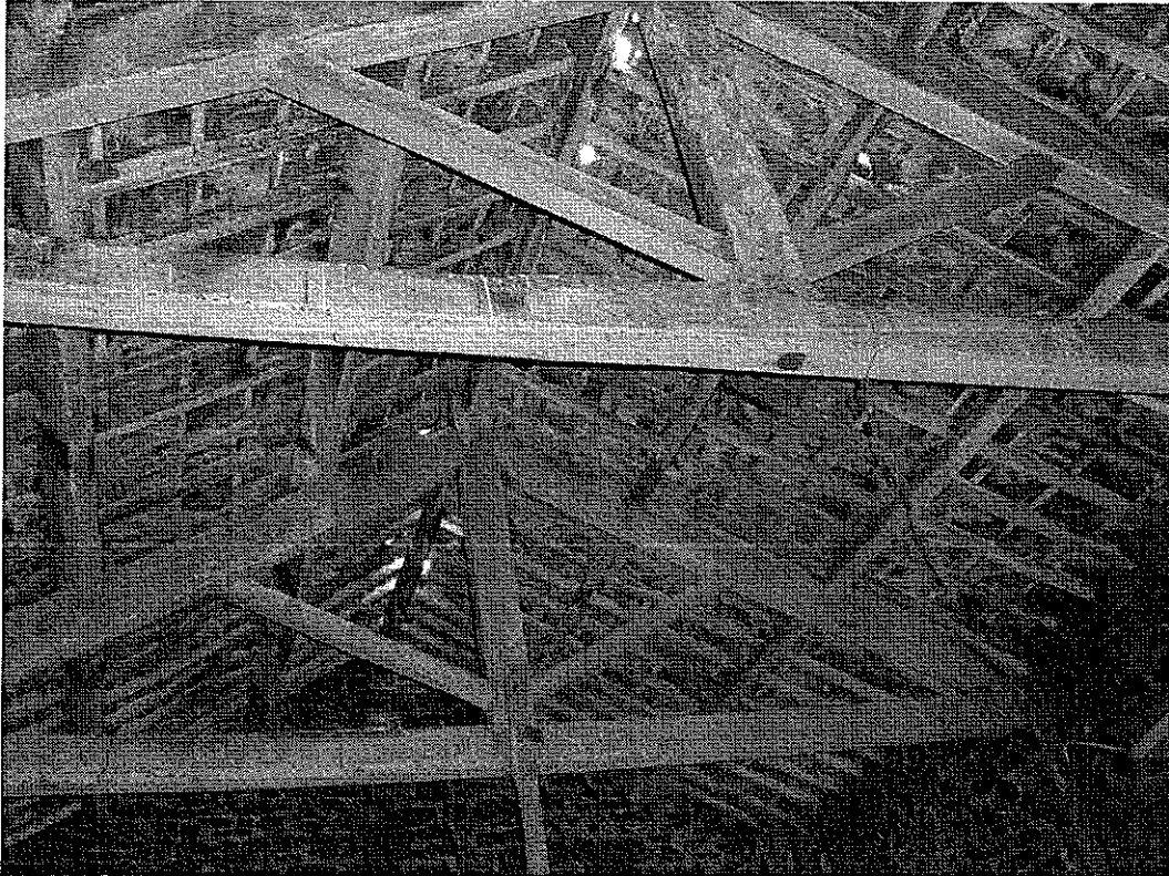
Barn Roof Showing King Post Trusses
