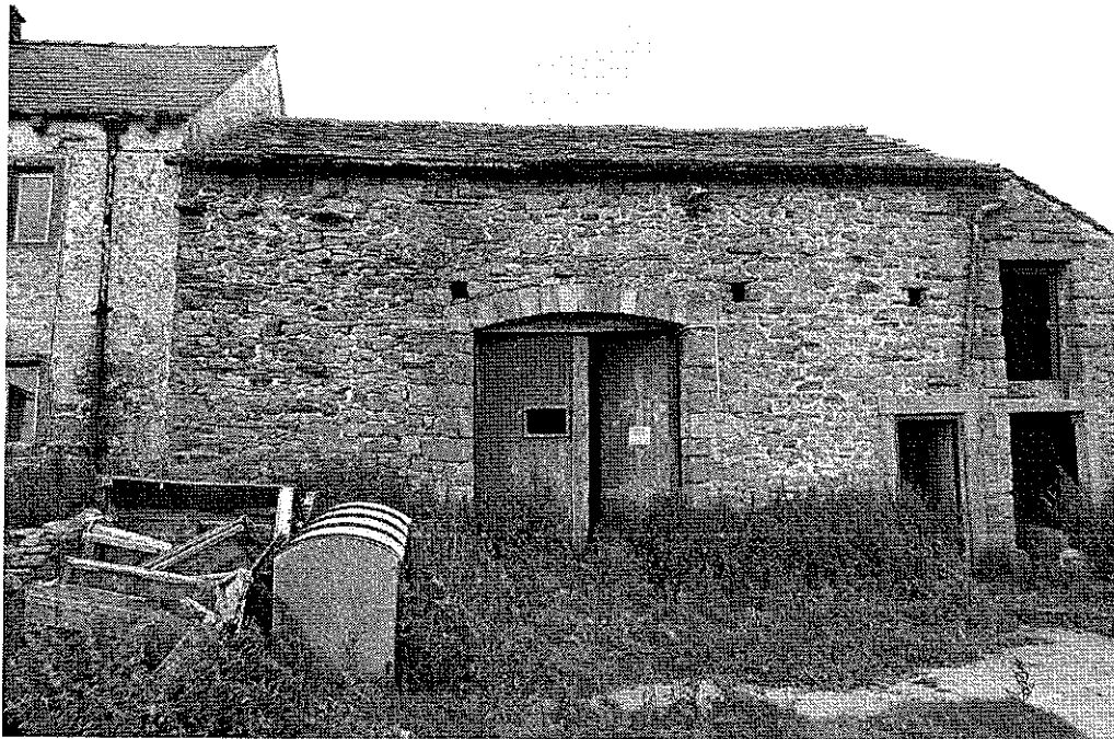
South East Elevation of Barn
