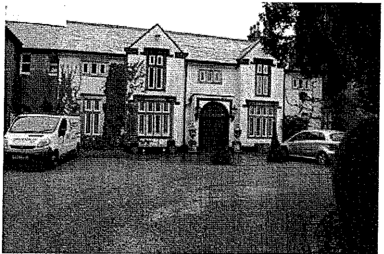
Photograph 2. The front of the function room block. The proposed porch would replace the doorway.
