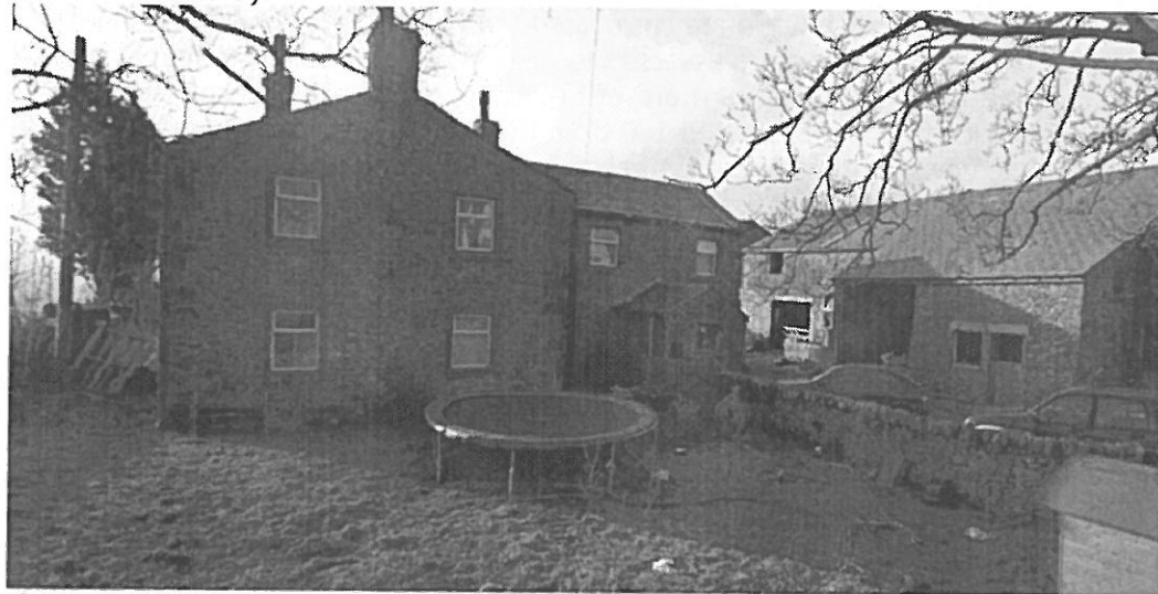
Photo 3: farm house to the left of shot and old barn to the right of shot
