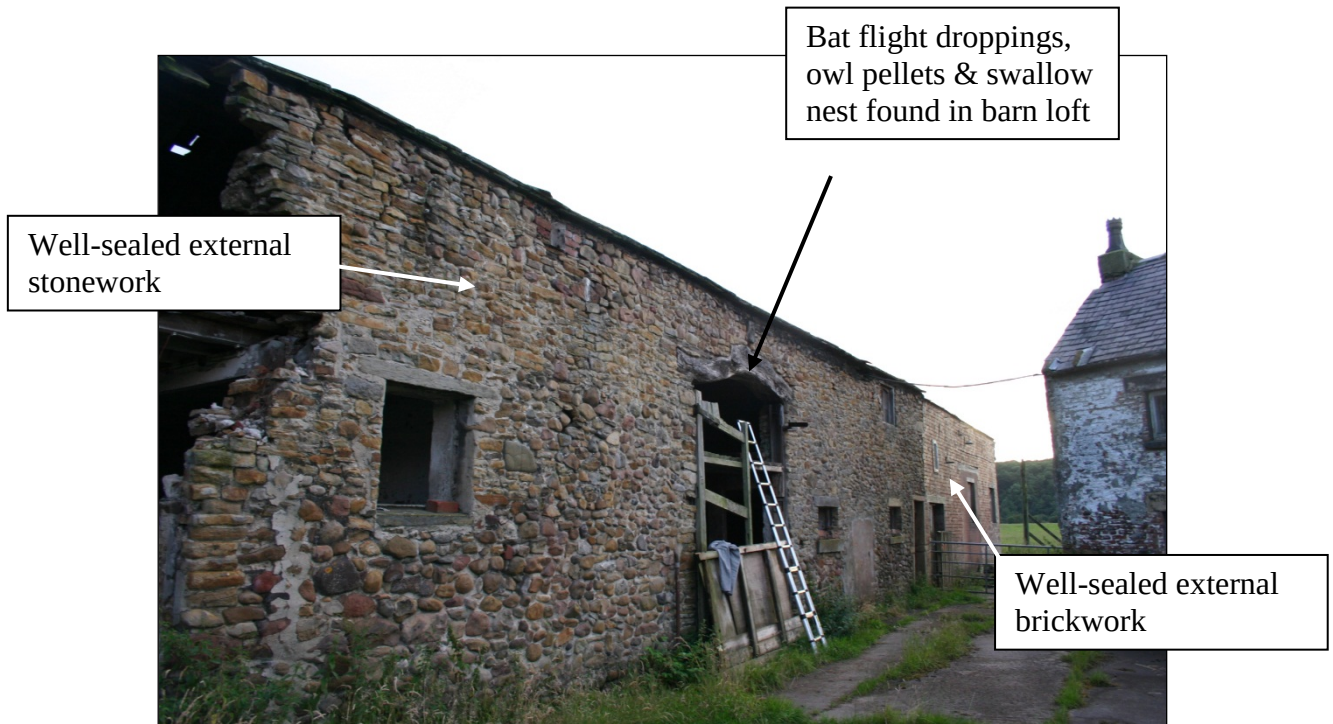
Plate 3. Eastern elevation of barn
