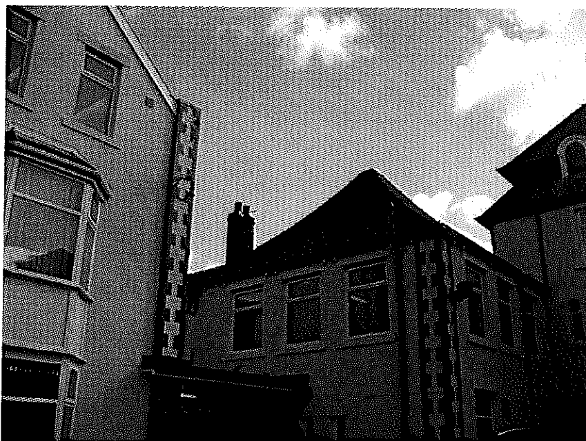
Photo 2 – Typical view of building on northern elevation
