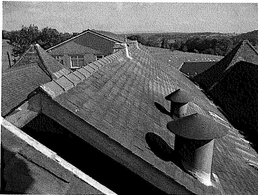
Photo 1 – View of multi pitched roof
