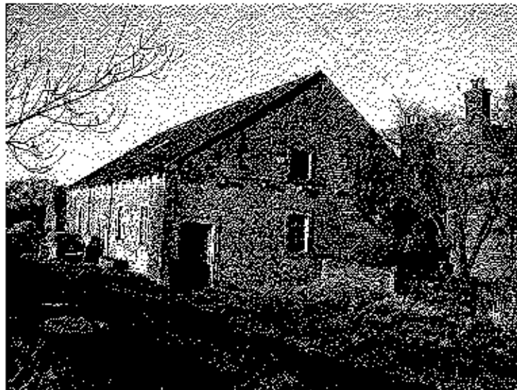
Image 03. Openings in wall of large barn facing North East. Note the oil tank will be removed. The large barn door opening will still be defined when windows are inserted to serve the ground floor. Barn B.
