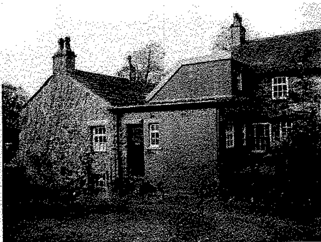
Rear elevation existing toilet extension
