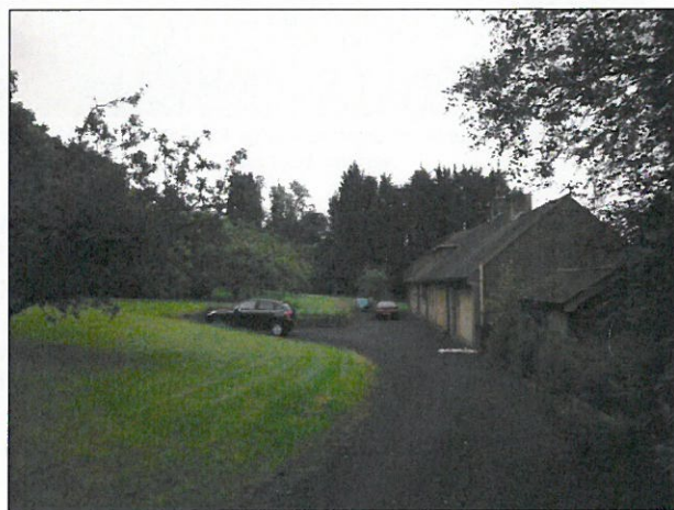
Fig. 2: The existing property, as seen from the west looking east, with group G9 in the background just right of centre
