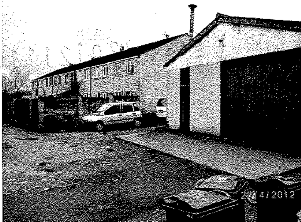
2. LOOKING WEST TOWARDS EXISTING TERRACE
