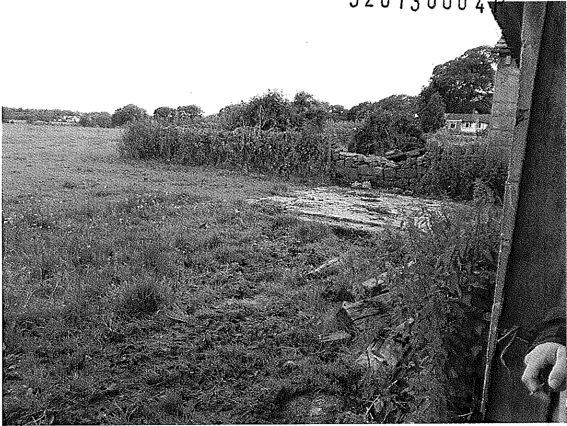
Photo 7 – External underground concrete slurry tank to W of site, looking NW.
