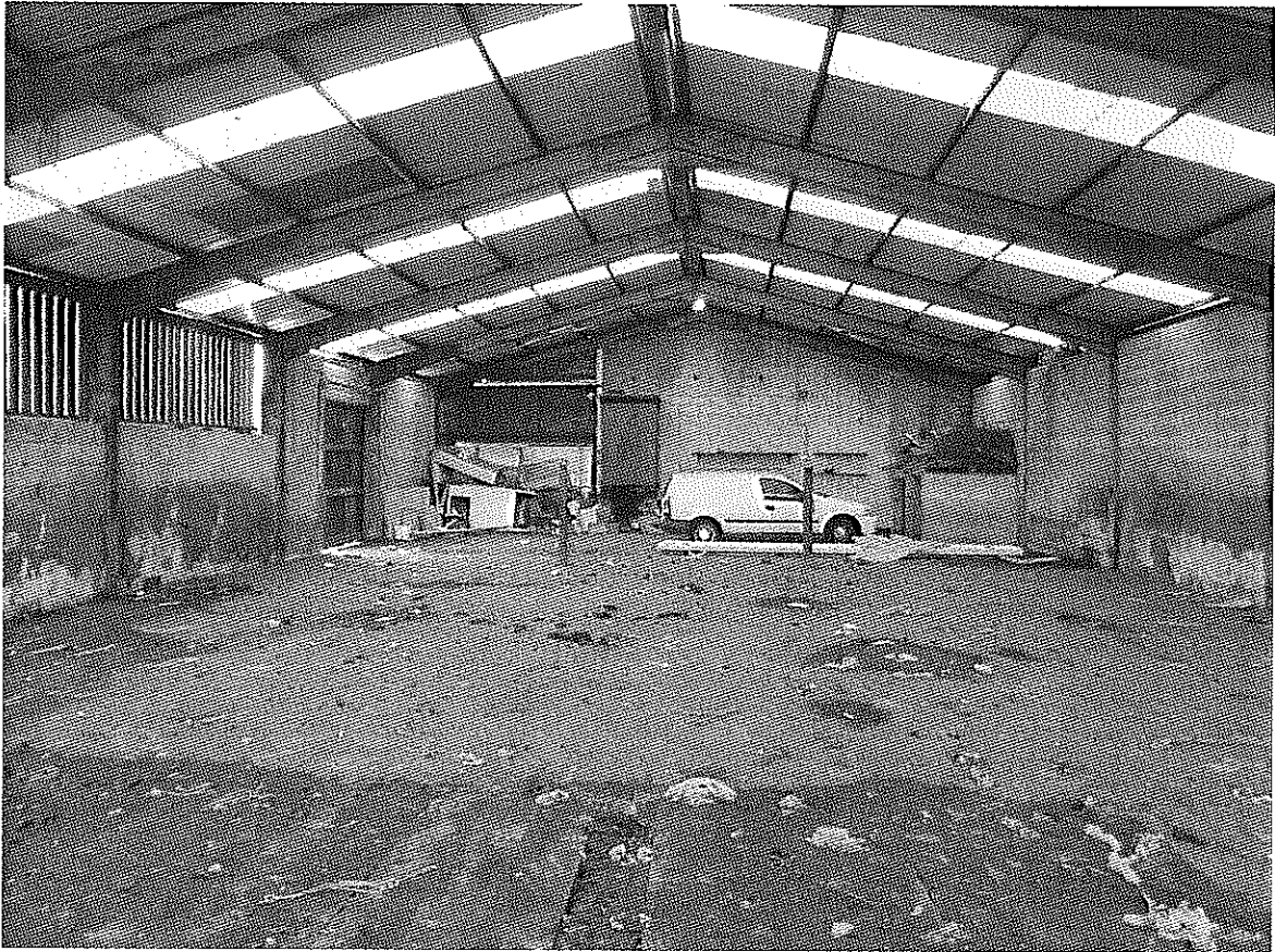
Photo 6 – Internal layout of building, looking NE, with concrete floor and metal/plastic roof. Some minor debris stored within barn.
