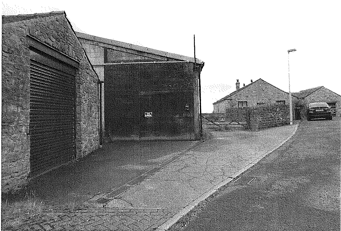
Photo 2 – NE elevation of barn with stone garage (foreground) to NE of site boundary, looking W.
