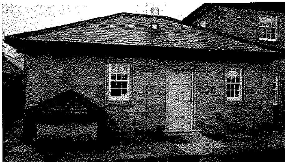
Front of the single storey outshot
