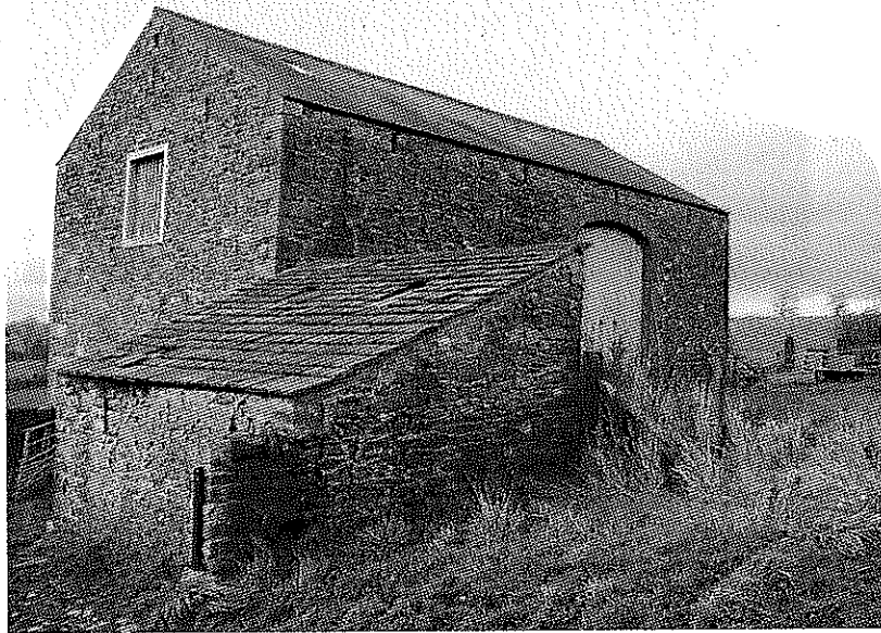
Photograph (3) – East elevation
