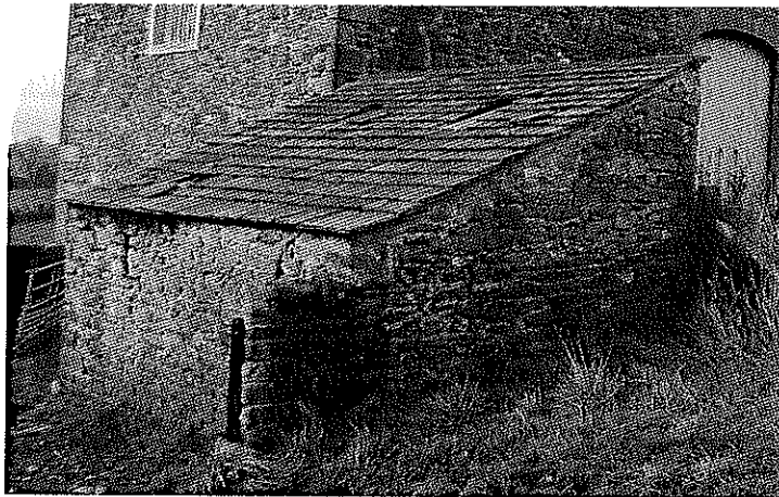
Photograph (1) – Outbuilding roof
