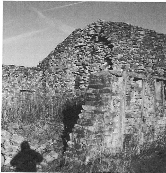
Photograph (14) – Showing the remaining internal skin of the random stone wall.
