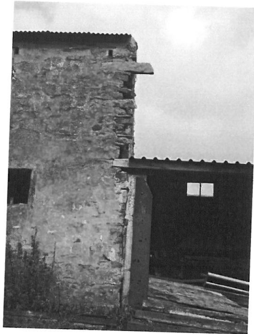
Photograph (2) – The cantilevering stones at the South West corner where previously this cottage would have been joined onto adjacent cottages.
