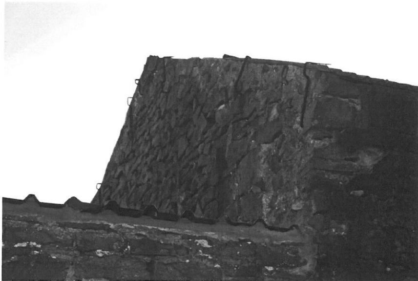
Photograph (6) – East Elevation showing the good condition of the stonework and the metal ties holding the corrugated roof sheeting in place.
