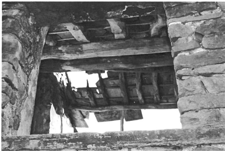
Photograph (21) – Showing part of the roof to the western cottage.
