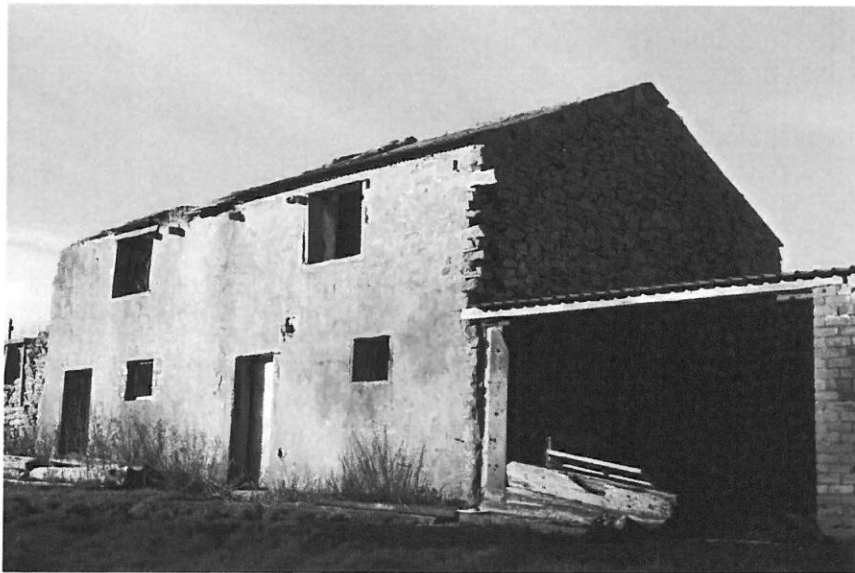
Photograph (7) – East Elevation showing the cantilevering stones at the south east corner as identified previously and the adjoining single storey outbuilding that is to be demolished.
