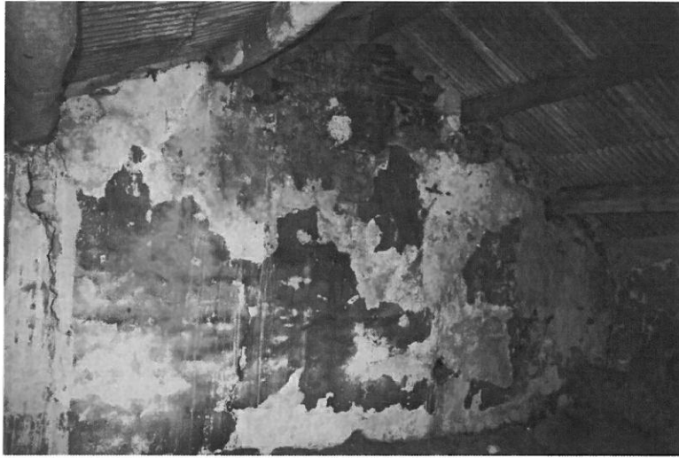
Photograph (22) – Showing the condition of the roof structure to the eastern cottage.
