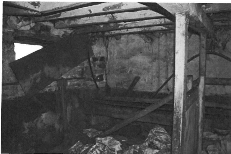
Photograph (18) – Showing the good condition of the walls and floor to the eastern cottage.
