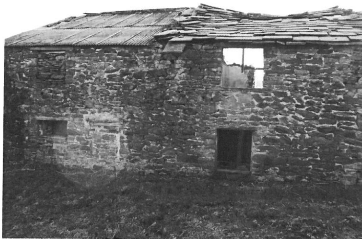
Photograph (20) – Showing the grey slate roof to the western cottage and the corrugated sheeted roof to the eastern cottage.
