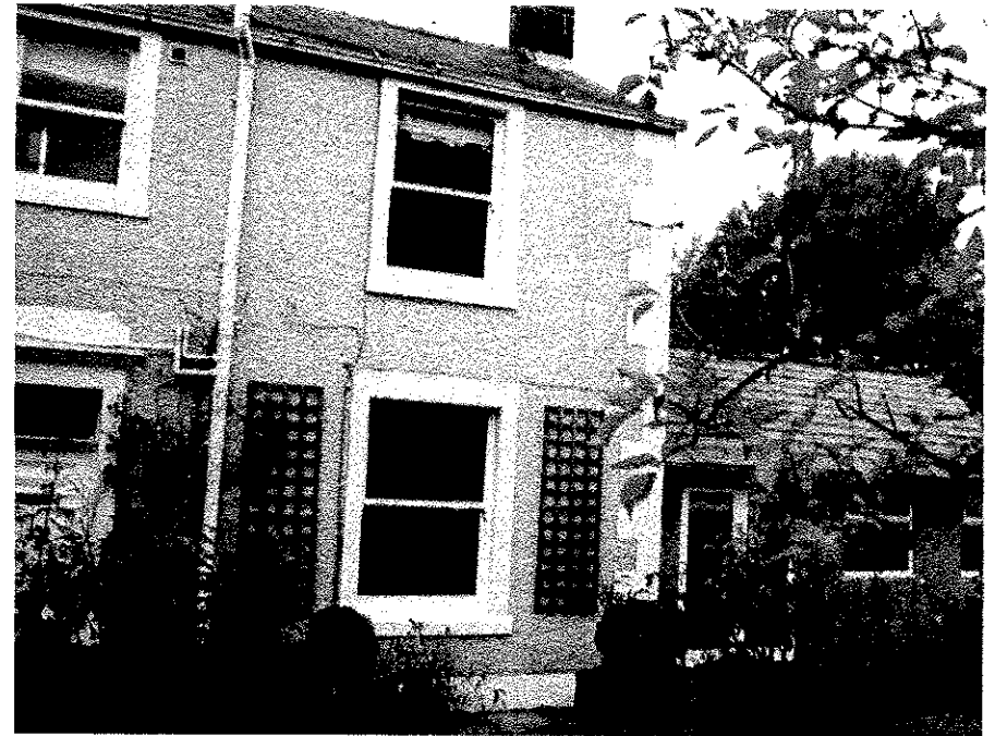
Main house & existing extension
