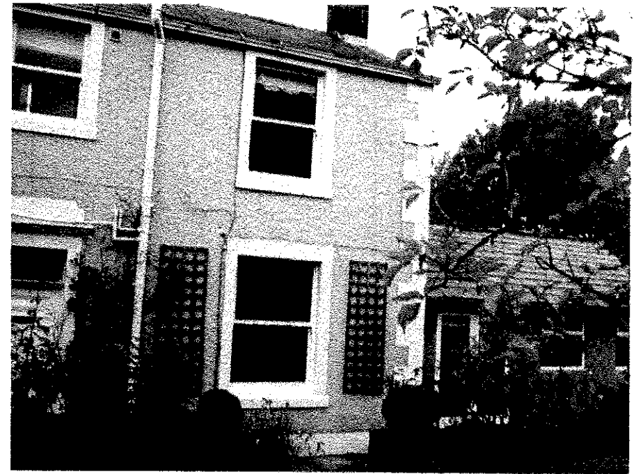
Main house & existing extension
