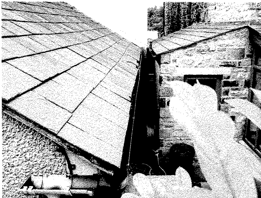
Back view to adjoining property
