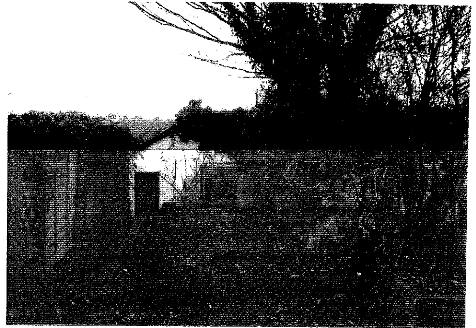
Removal of garage and tree creating new access and parking area
