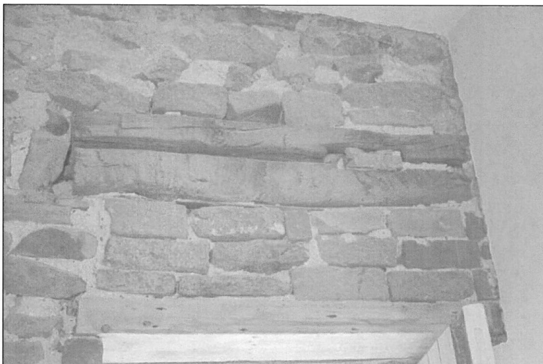
18. Fragment of rail in rear wall above doorway, possibly originally reused as window lintel
