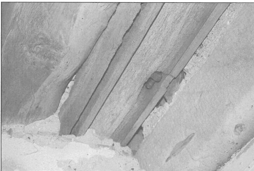
19. Re-used timber door jamb, gudgeon pin remaining, now inner lintel of front window
