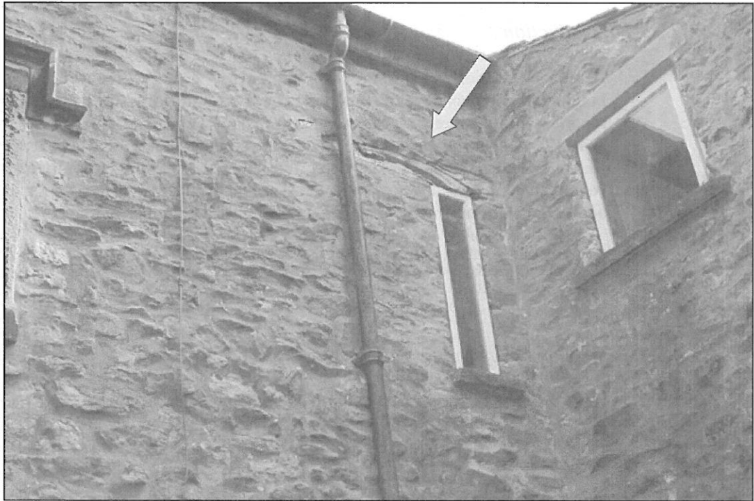
4. Rear of Number 3 Abbeycroft showing timber which may be former wallplate, suggesting possible timber-framed origins and the heightening of the building during its cladding
