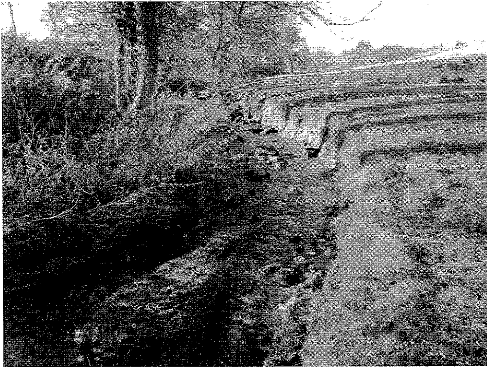
Photograph 8: Section showing typical conditions where no constraint to survey occurred.
