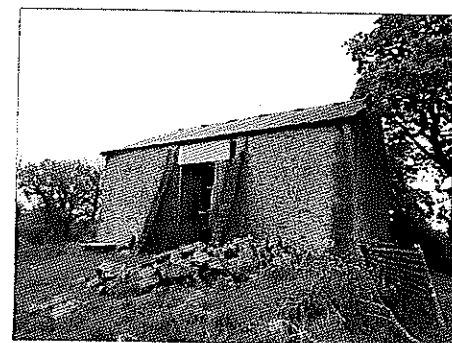
Photo F: Building 7
