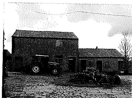
Photo B: Building 1 (north elevation)
