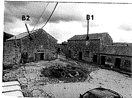
Photo C: Building 1 (north elevation) and Building 2 (west elevation)
