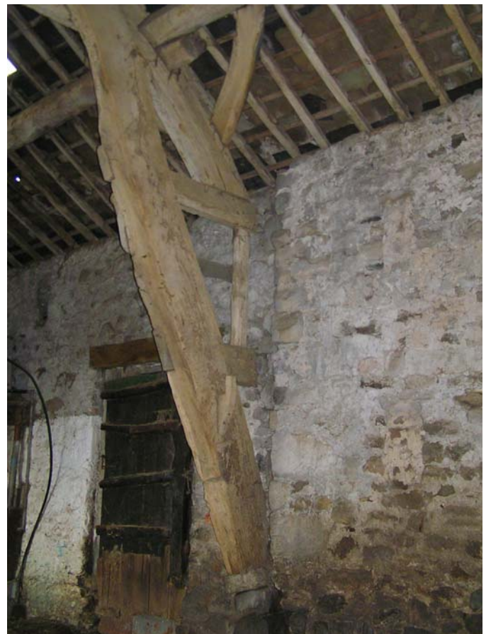
Detailing of the cruck
