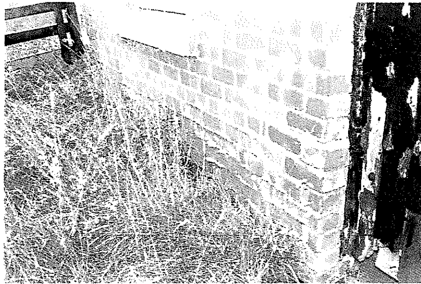
PHOTOGRAPH 6: VIEW OF NORTH WESTERN EXTENSION TO THE BARN WHERE IT MEETS THE BANKING
