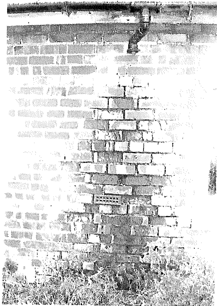
PHOTOGRAPH 5: VIEW OF THE WATER DAMAGED SECTION OF THE SOUTH EASTERN ELEVATION WALL
