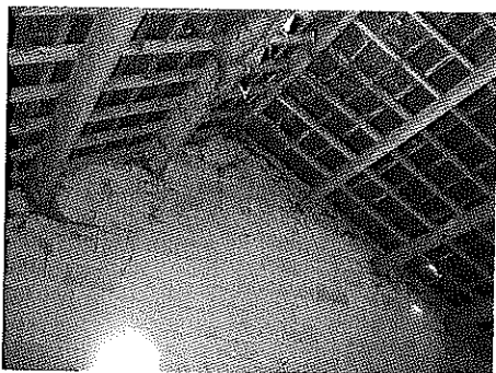
Figure 8: Barn B - roof detail
