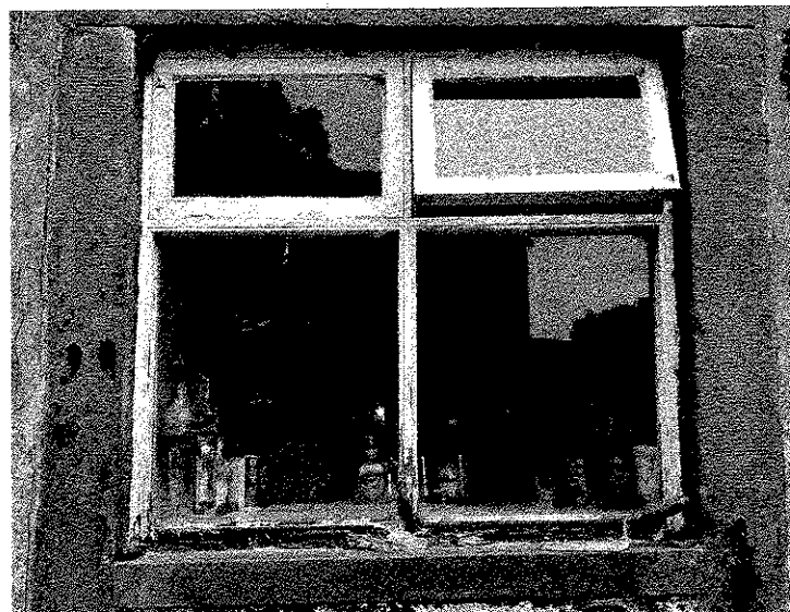
Casement timber window frames to north west and north east elevations.
