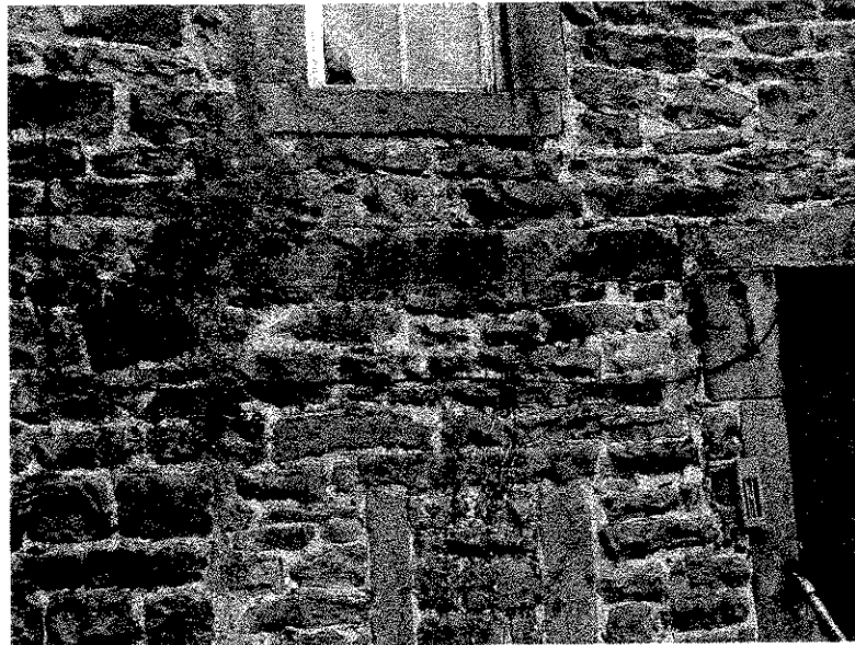
Infilled stonework - dressed stone surrounds (bottom centre)
