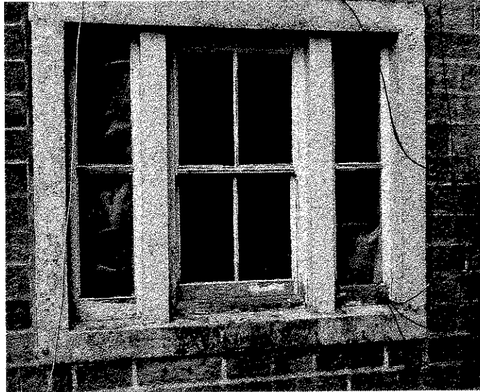
Traditional sliding sash timber window frames to the south west elevation and north west elevation (Kitchen).
