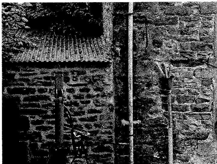
Profiled sheeting to attached outbuilding on south east gable
