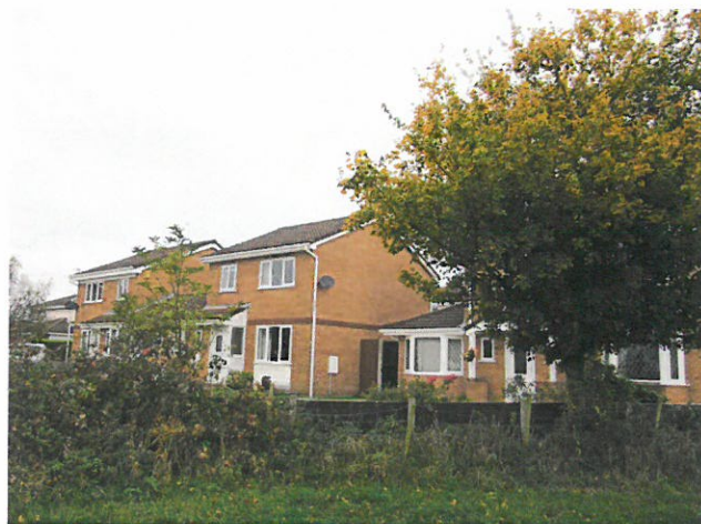
PHOTOGRAPH 11 view of properties on lindale road facing the site
