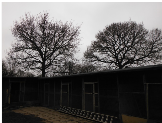
Fig. 2: Kennel buildings inside the site, looking west, with Oak trees T6 (right) and T7 (left) visible to rear
