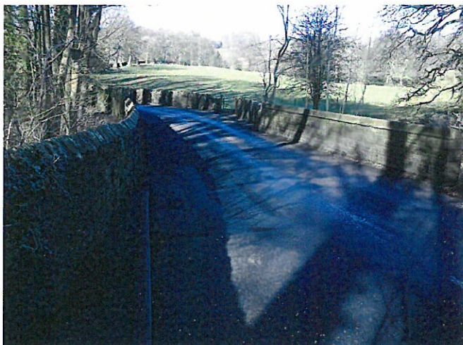
Photo B5; Existing bridge on Whinns Lane within the double bends
