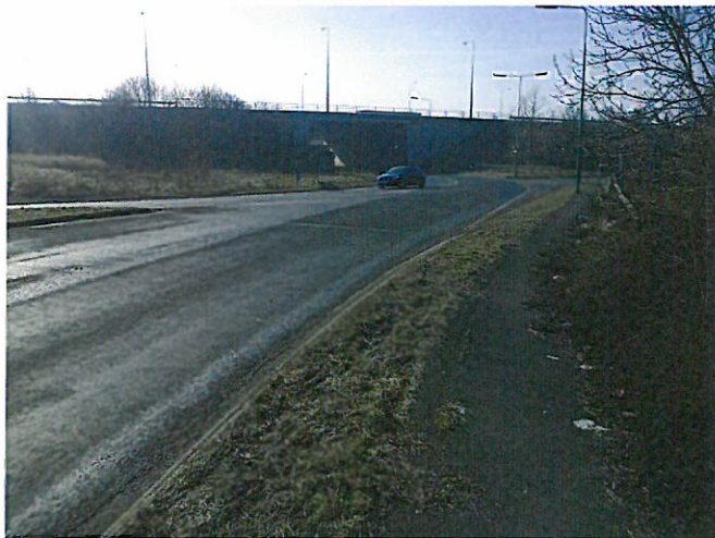
Photo B3; A6068 exit from M65 junction 8
