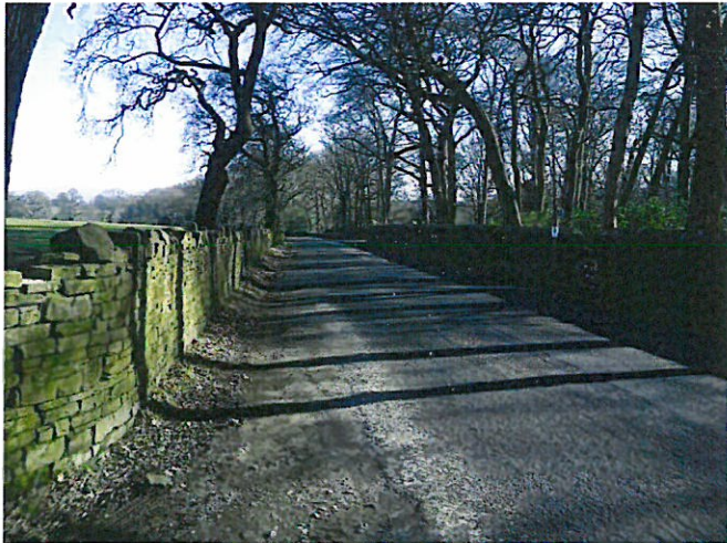
Photo B3; Visibility to left from carriageway edge at proposed site access
