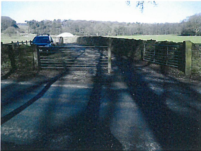
Photo B1; Huntroyde Farm track access from Whinns Lane, showing double gates with removable centre pillar
