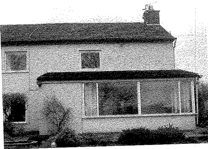
Rear lean - to, to be demolished.
