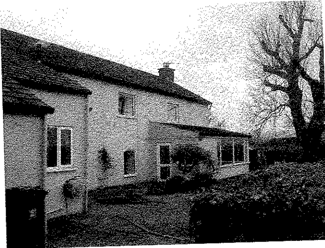
Rear West facing elevation.
