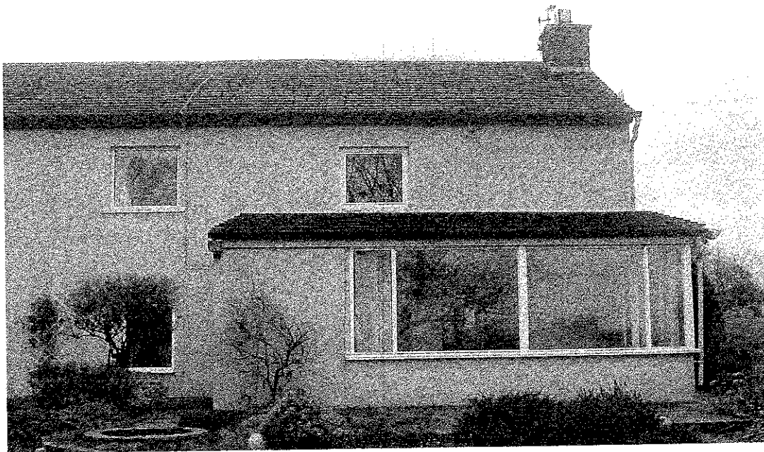
Sun room extension which is to be replaced with a garden room.
