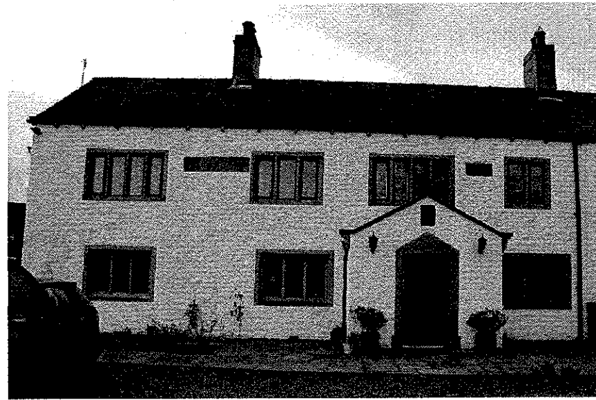
Photograph 4 NE elevation Edisford Hall Farmhouse.
