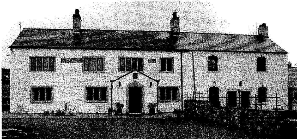
East elevation (rebuilt c.2006)
