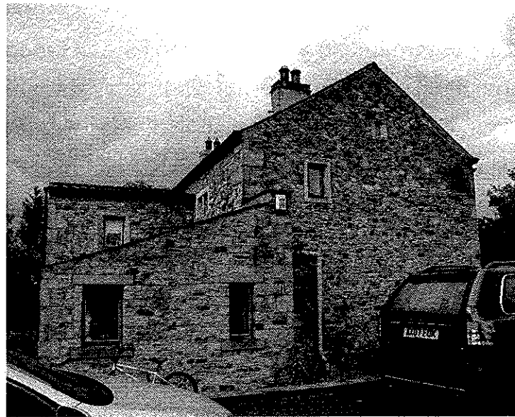
Photograph 6 SE elevation Edisford Hall Farmhouse.
