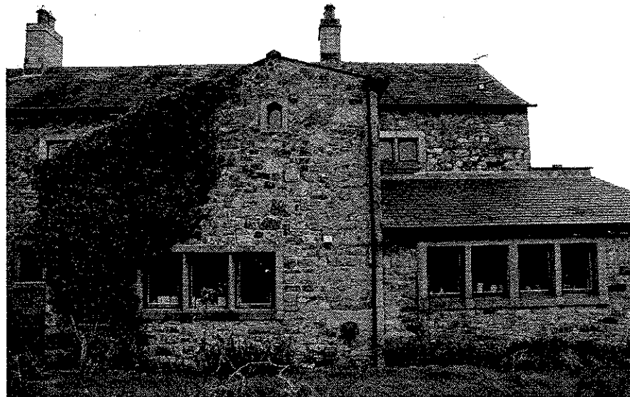
Photograph 5 SW elevation Edisford Hall Farmhouse.
