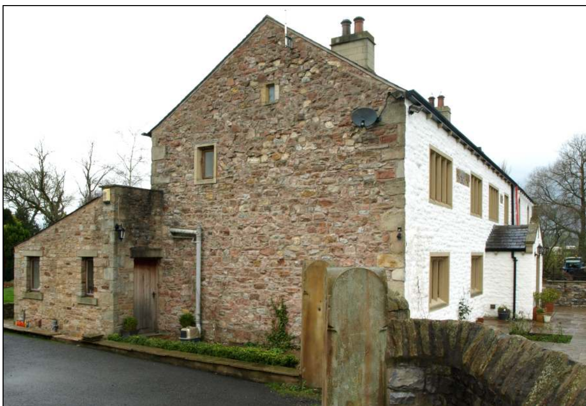
Photo 2: South gable, with part of 1984 extension at left
