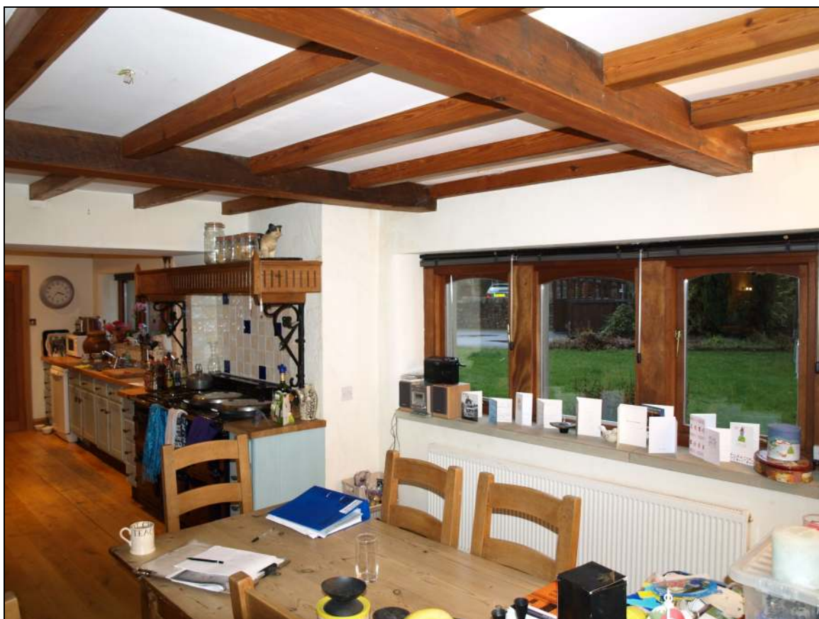
Photo 4: Interior of kitchen within wing (former site of stairs), and 1984 extension beyond (far left)
