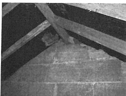
Figure 5: south-west gable apex wall
