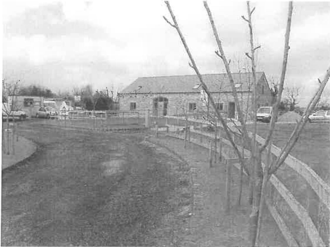
Fig 3 - Photo of adjacent dwellings (Roadside Farm Barn and Roadside Farm Cottage)
