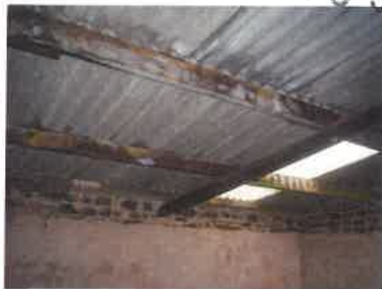
Machinery/cattle store roof.
