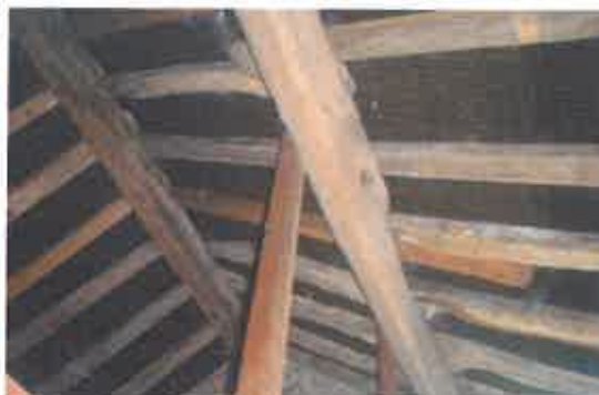
The farmhouse roof voids
