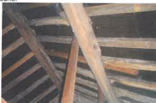
The farmhouse roof voids
