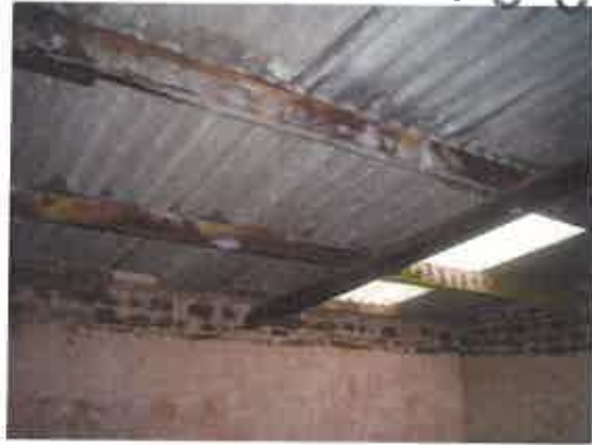
Machinery/cattle store roof.
