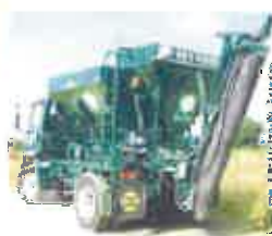
Typical paving machine in use.
