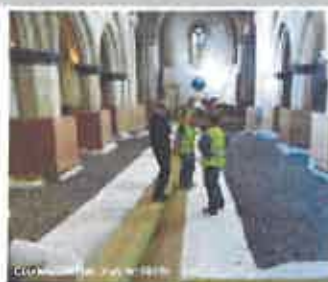
Two workers laying out the Ty-Mawr insulated limecrete floor
