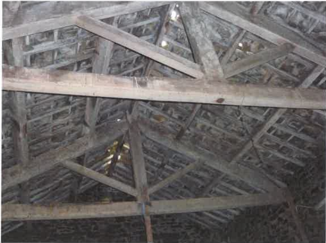
Barn Roof Showing King Post Trusses
