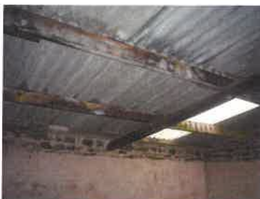
Machinery/cattle store roof.
