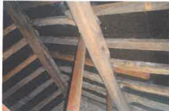
The farmhouse roof voids
