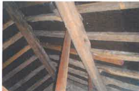
The farmhouse roof voids
