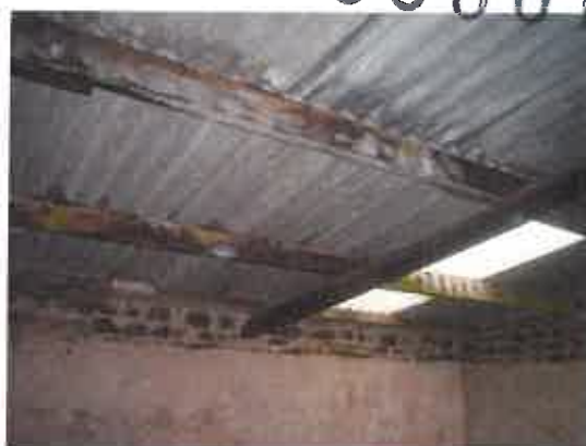
Machinery/cattle store roof.
