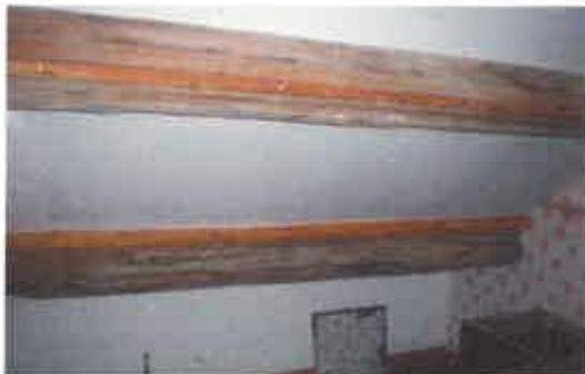
The roof space in the cat slide roof.
