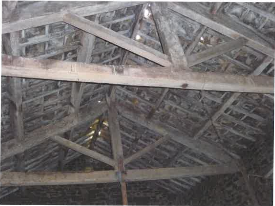
Barn Roof Showing King Post Trusses
