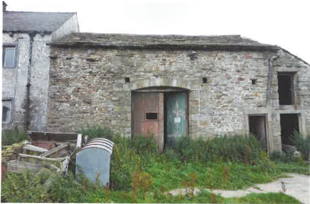
South East Elevation of Barn
