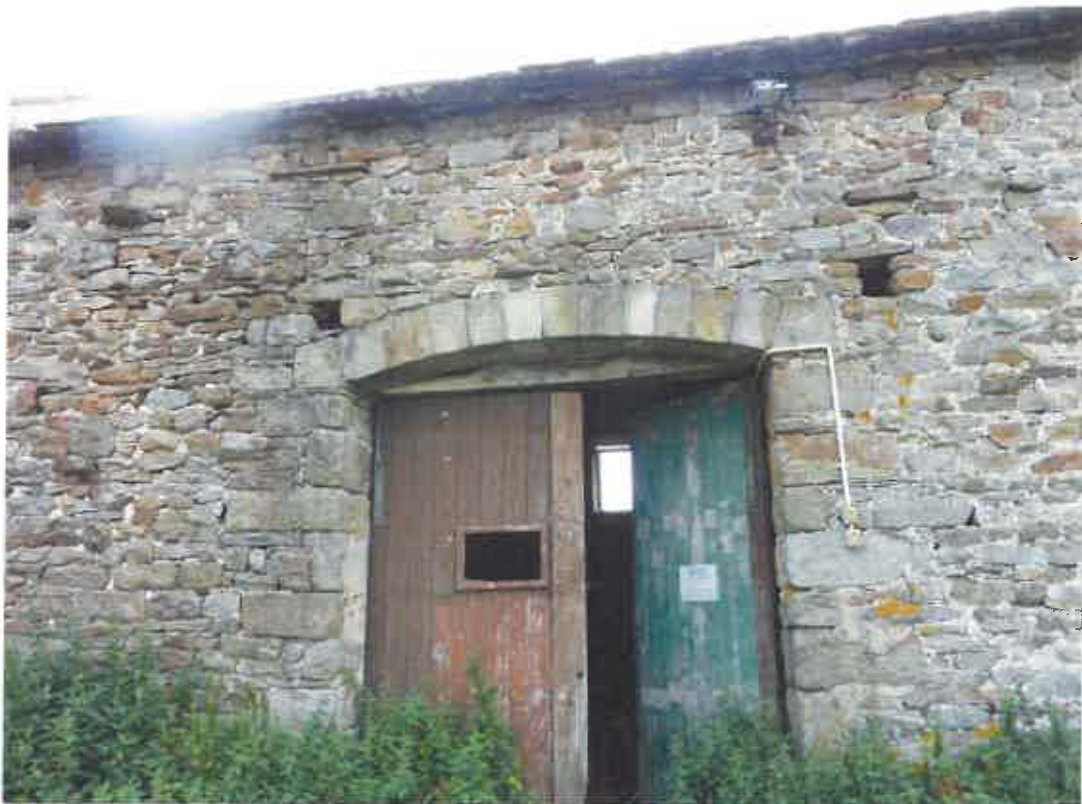
Barn entrance, details of random stone and the general sound condition of the building.
