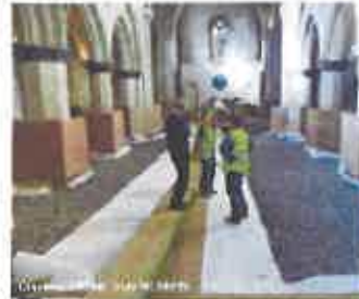
Rebuilding the floor at Chester Cathedral
