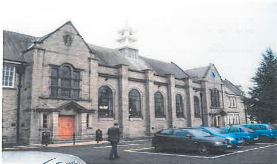
View of the existing elevation featuring the 5no identical windows to be replaced as can be seen between the two protruding entrance areas.
