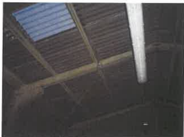
Stable/ store roof
