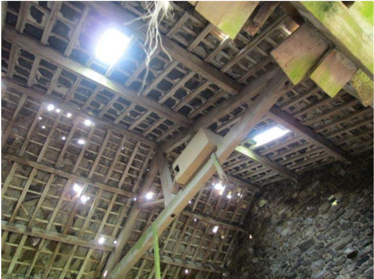
Image 5: Internal view showing roof condition
