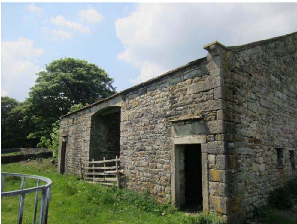
Image 2: Rear Elevation – South facing
