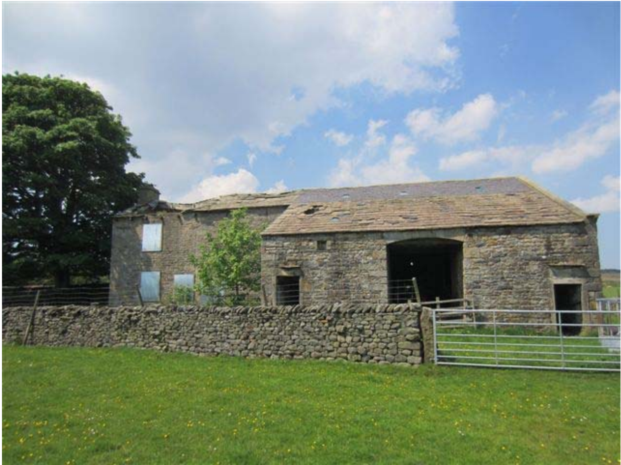
Image 1: Rear Elevation showing boarded up windows and well defined existing curtilage
