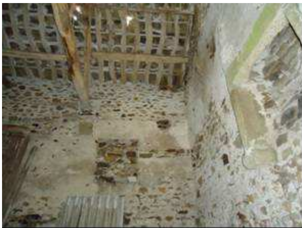
Image 2 – Partially lime rendered walls and mortar work in good condition.
