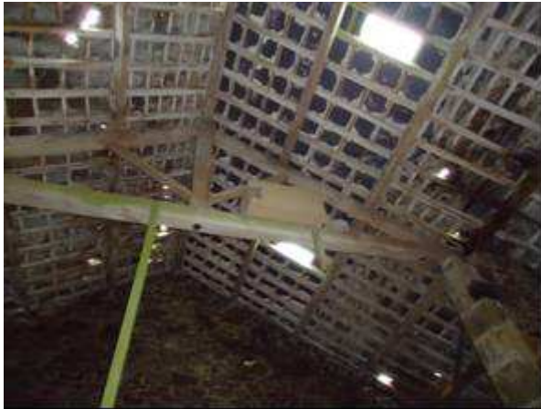
Image 1 – Interior of the barn, showing the roof structure and location of the barn owl nesting box.
